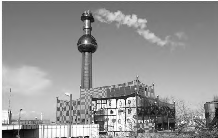
FIGURE 11.2. Hundertwasser garbage incinerator, Vienna 1987: hiding a power plant by “oratory in architecture.”
